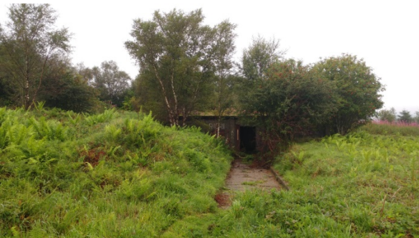
Before Groundwork and Grills Fitted
